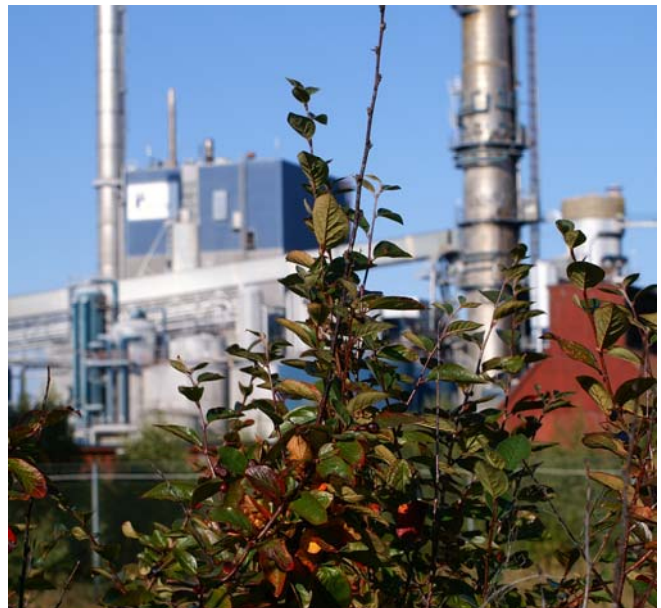
Vallvik Mill and its soda boiler and digester
